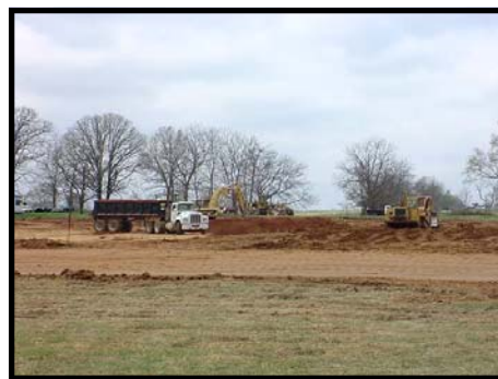
Crews began initial groundwork last week on the building site.
